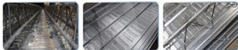
“M”型钢筋桁架楼承板局部特写
